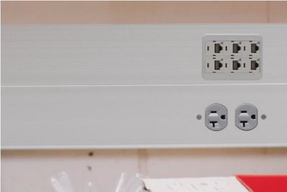
Prewired Raceway
