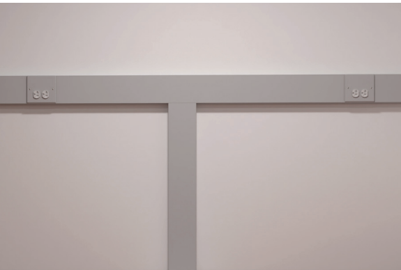
Prewired Raceway
