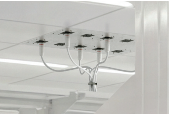
Multi-Service Electrical Ceiling Panel
