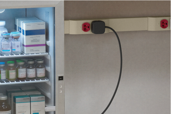
Plugmold with Hospital Grade Receptacles
