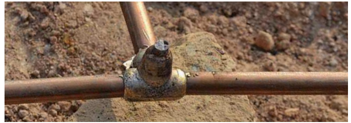
TA nVent ERICO Cadweld connection
