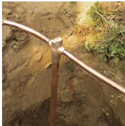
GT Cadweld connection
